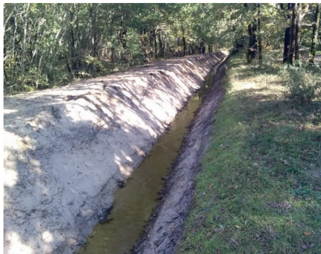
Reprofilage fossé, Lège-Cap Ferret
