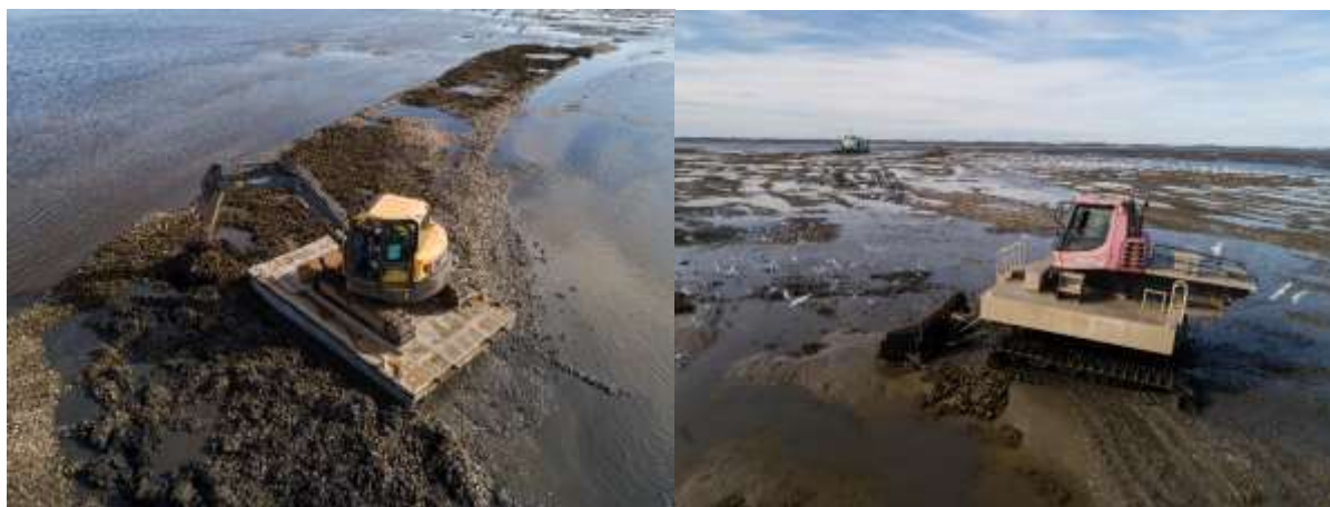
Figure 5: Illustration des travaux
