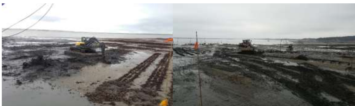
Figure 2: Illustration des travaux
